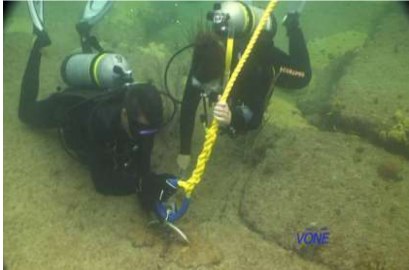
Figure 4: Volunteers from Vone Research, Inc. attaching a new mooring buoy to an anchor.
